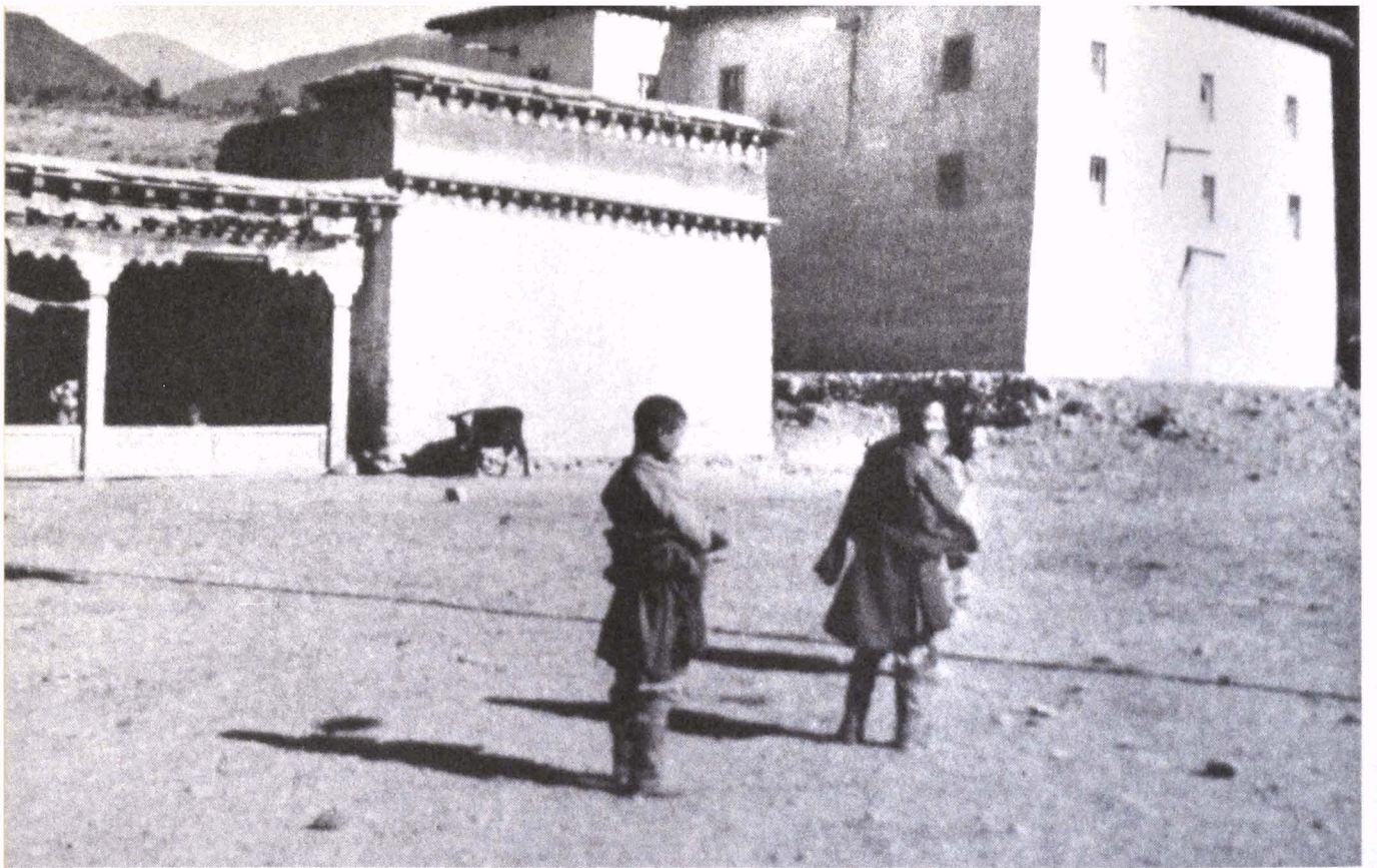
Pangdatshang's house in Bo, with a family temple on the extreme left. The wooden channels projecting from the wall of the house on the right are part of the primitive plumbing system and carry away the waste water.
